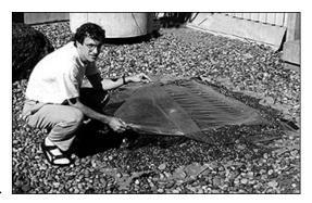
the pit. Two layers are used in case one develops a small leak. Use inexpensive polyethylene, although special UV- stabilized plastic will last longer.
